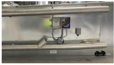
The Solution: Carolina Heat Pipe's "St Mach 1 TRAHP™" (Thermosyphon Run Around Heat Pipe) System. The TRAHP™ is a matched pair of refrigerant charged heat pipe coils positioned around the cooling coil. The "precool" coil absorbs heat energy from the incoming / return air and transfers this energy to the "reheat" coil downstream of the cooling coil. This warms cold saturated air leaving the cooling coil to provide to dehumidified supply air.
