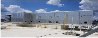
The heat pipe requires minimal maintenance of periodic coil cleaning for the life of the air handler.
